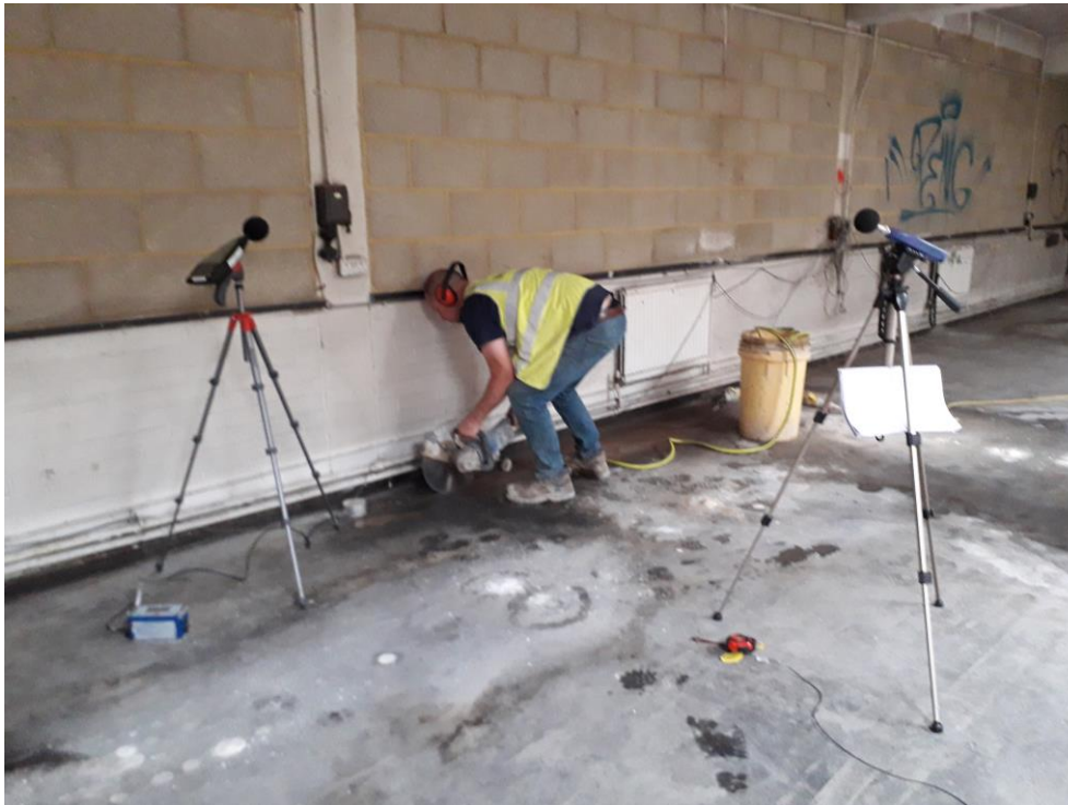
A3.12: Test No. 12 – Saw cutting Slab, Main Room, First Floor.
